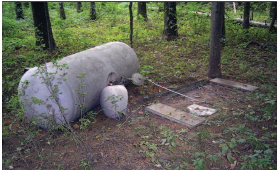
Figure 5W-5. An improperly anchored tank; tethered only by a supply line
