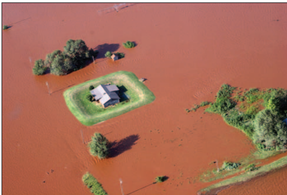
Figure 1-12. Home protected by a levee
