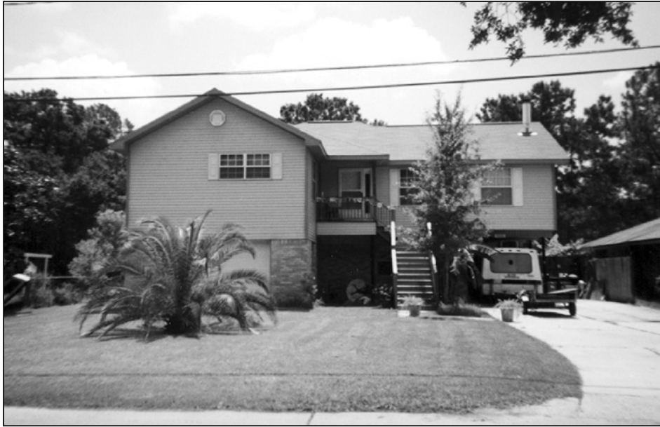
Figure 1-2. Elevation of existing residence on extended foundation walls
