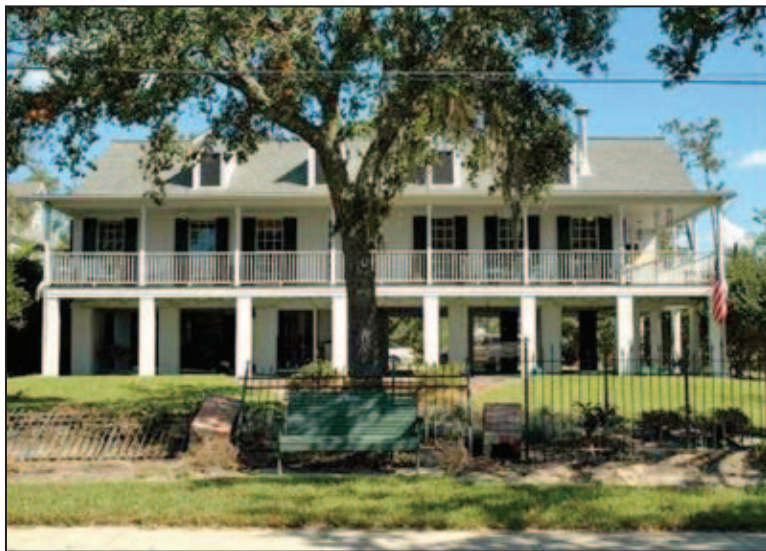
Figure 6-29. Elevation on timber piles
