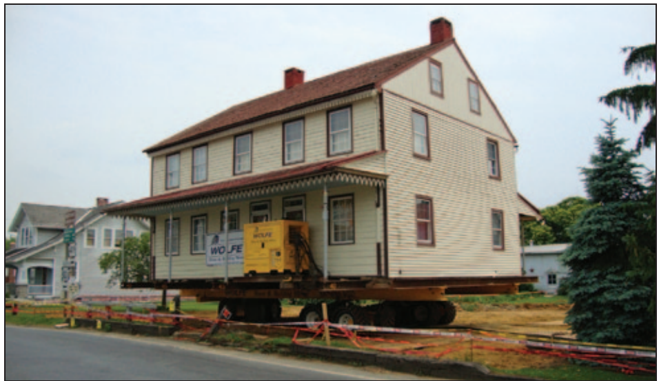
Figure 5R-12. Trailer is used to pull the house to the street (photo courtesy of Wolfe House Movers)
