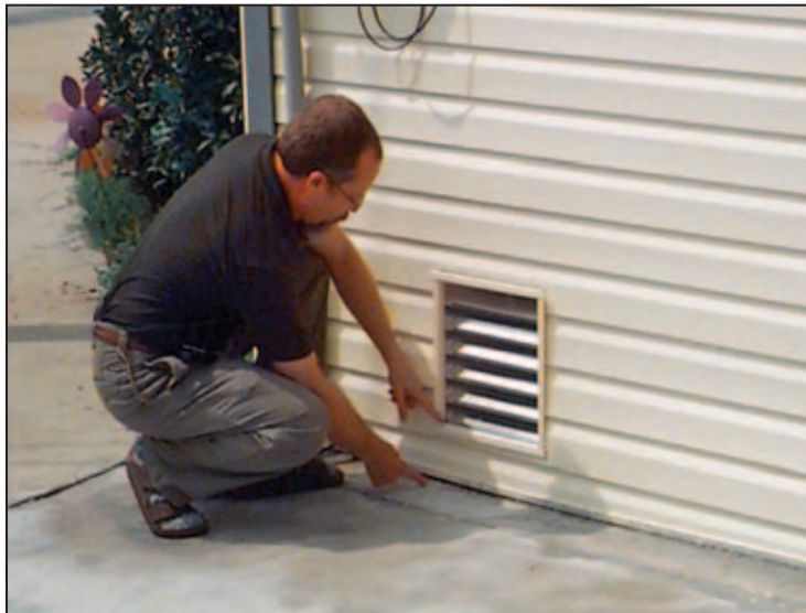
Figure 6-43. Example of flood vents
