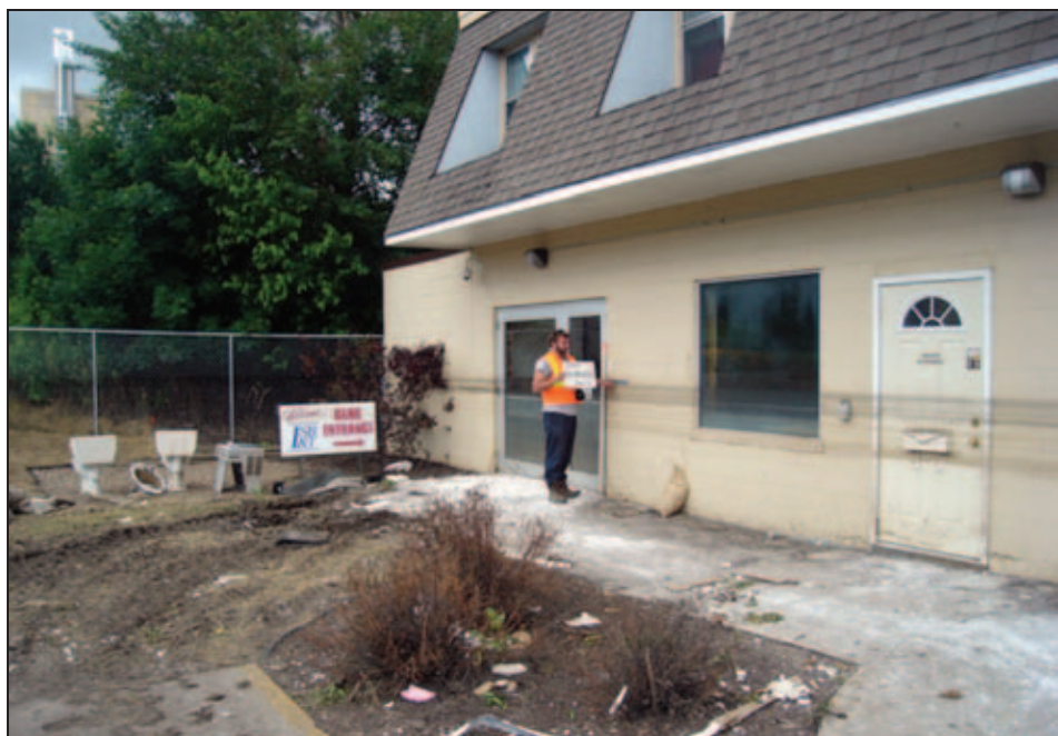
Figure 3-6. Measuring mud lines or high water marks to establish flood depth
