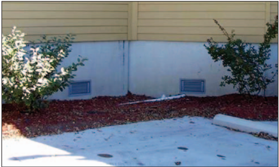
Figure 6-42. Example of flood vents
